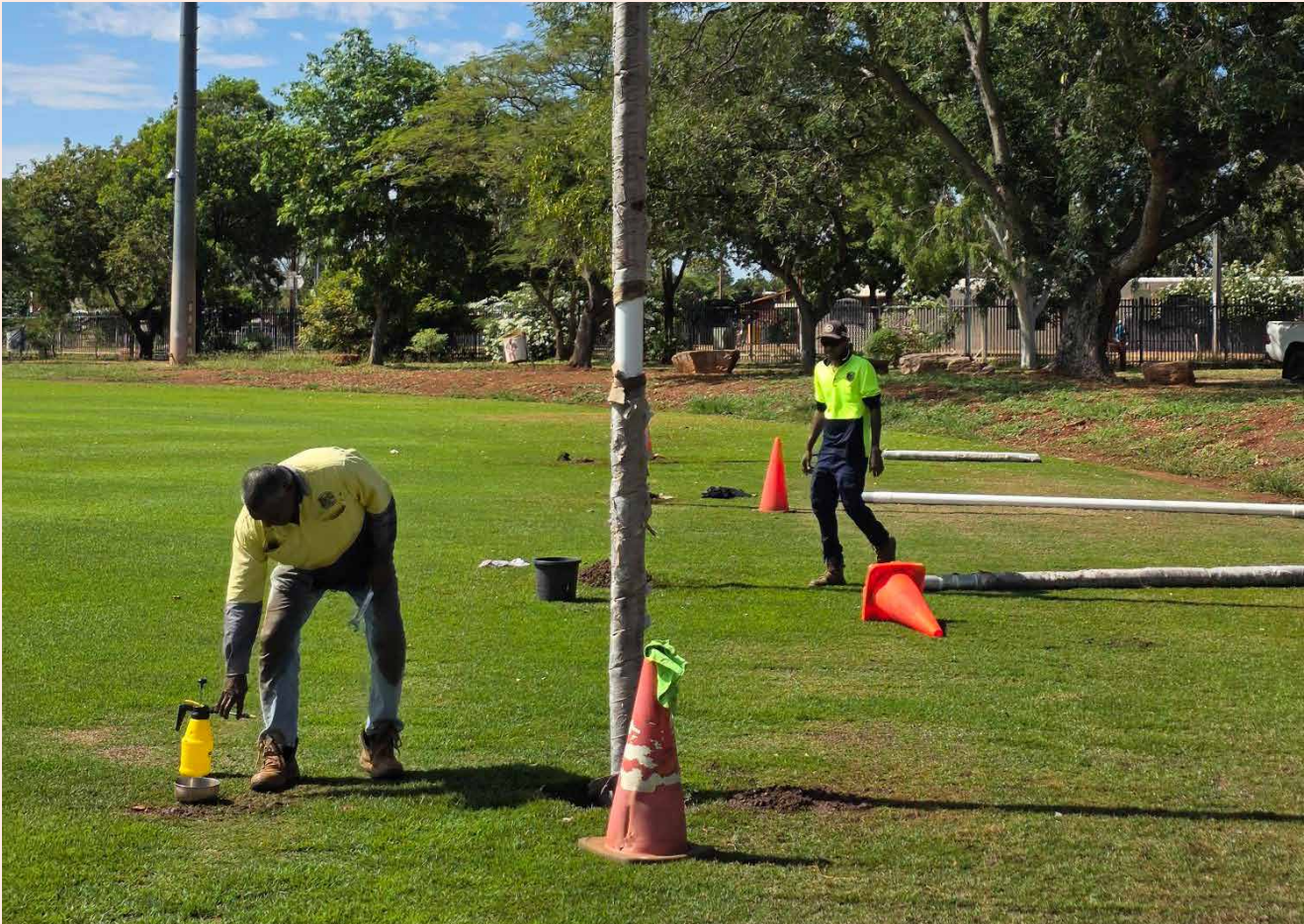
Preparing the new Halls Creek oval. Credit: Shire of Halls Creek
